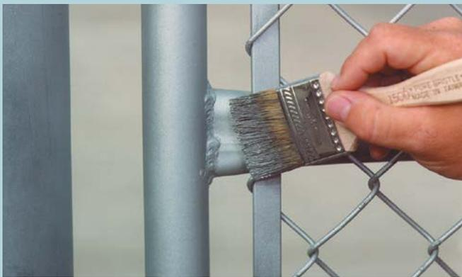
One commonality of all zinc coatings examined thus far is the cathodic protection afforded. Zinc-rich paint coatings are different than the other coatings as there is a binding material used to adhere the zinc particles. For cathodic protection to be possible, the zinc dust must be at a concentration high enough to provide for conductivity between the zinc particles and the steel. This
