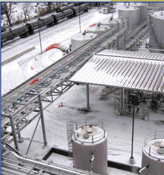
The exposed galvanized steel used in this plant will be protected from harsh snow and rain exposure.
