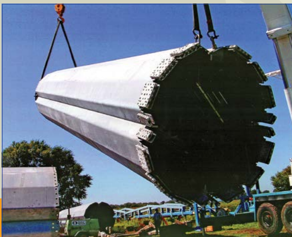
Separating the wind tower into several pieces made it considerably more economical to transport.
