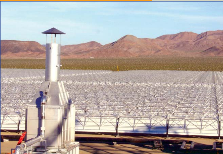
This solar energy farm is the largest capacity facility of its kind built in the past 15 years, spanning more than 400 acres with computer-controlled reflective mirrors.
