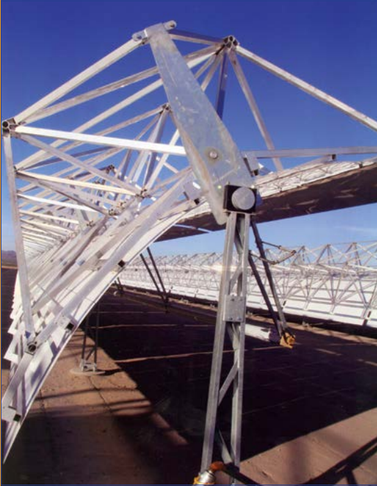
Located in the sun-drenched deserts of Nevada, the Solargenix Energy project harvests solar energy.
