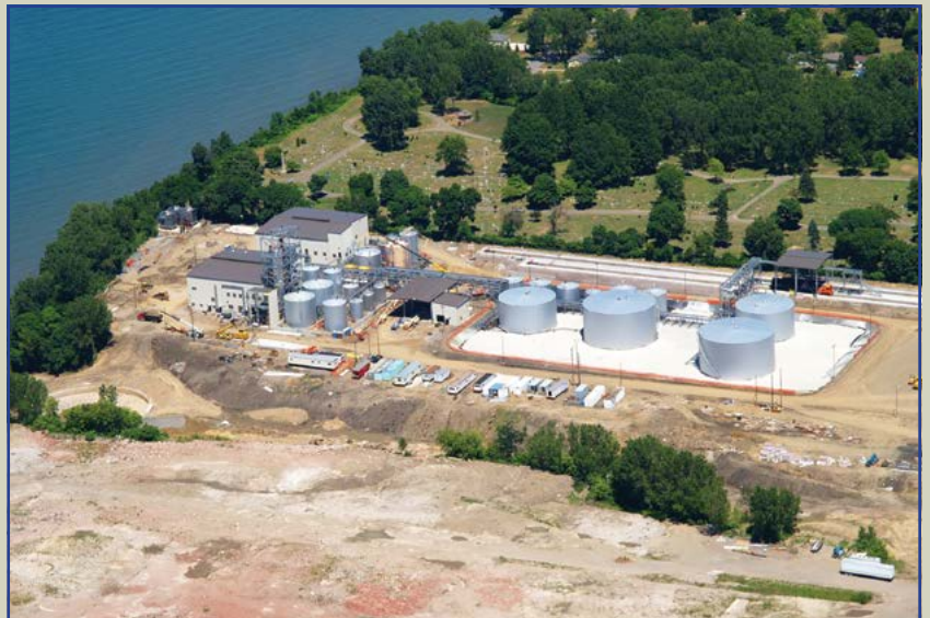
Located in an area where the biofuel industry is booming, the Lake Erie Biofuel Plant is designed to produce 45 million gallons of biodiesel each year.
