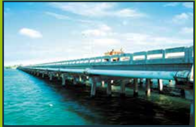
Boca Chica Bridge in Florida
