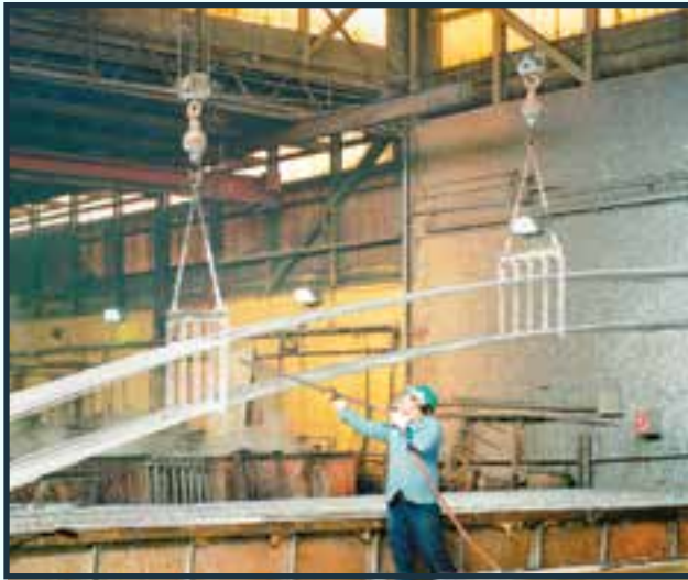
Removal of galvanized rebar from the zinc bath
