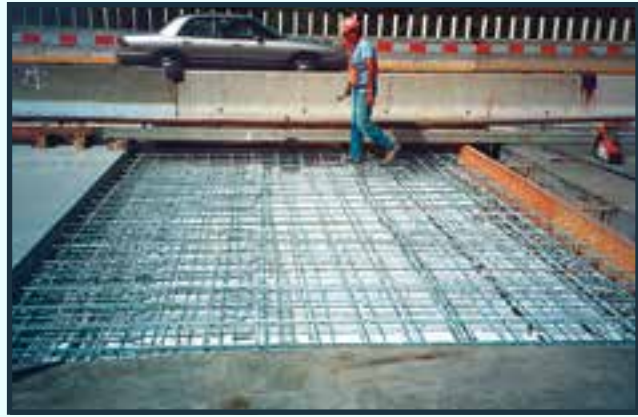
Because of its unique, tough coating, galvanized steel requires no special handling at the work site.
