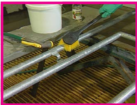
Organic contaminants can be removed using alkaline or acidic solutions, or solvent cleaning.
