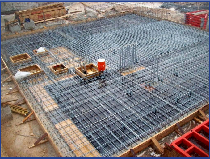
Magistrate Court and Hamilton Police Station in Bermuda utilizes hot-dip galvanized reinforcing steel to combat the corrosive tropical environment. All infrastructure in Bermuda requires hot-dip galvanized rebar.
