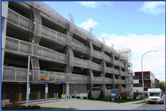
The Cincinnati Children's Hospital Parking Garage uses a combination of hot-dipped galvanized and stainless steel to create an aesthetically appealing exterior façade. The "ribbons of steel" design will remain beautiful for patients and medical staff well into the future.
