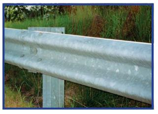
The zinc patina on a piece of fully weathered steel, seen left, will create a more successful duplex system when left on the surface.
