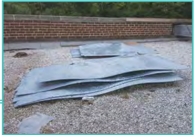
FIGURE 17: DISTORTION (ACCEPTABLE)
