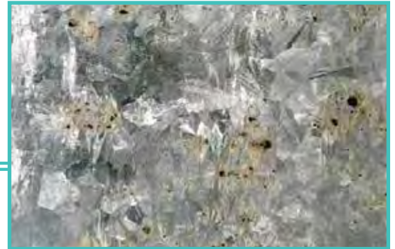
FIGURE 20: EXCESS ALUMINUM IN GALVANIZING BATH (REJECTABLE)
