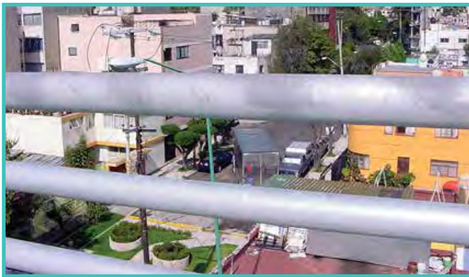
FIGURE 11: GRAY COATING DUE TO PROCESSING (ACCEPTABLE)
