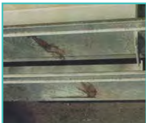
FIGURE 34: WELDING BLOWOUT (REJECTABLE)
