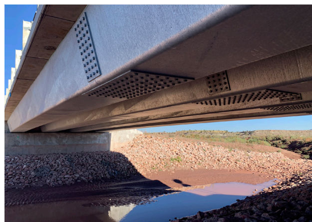
PRESS BRAKE TUB GIRDER BRIDGE
