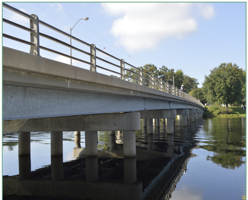
STEARNS BAYOU BRIDGE
