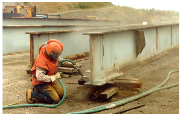
FIGURE: BLASTING BEFORE HDG
