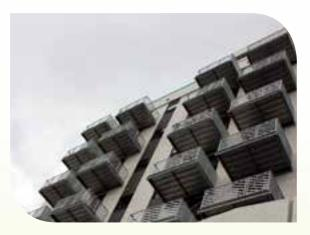
...the hot-dip galvanized balcony reduces the total cost over the life of the structure by 96%.
