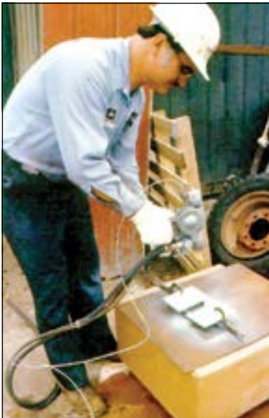
Zinc Spray Metallizing
