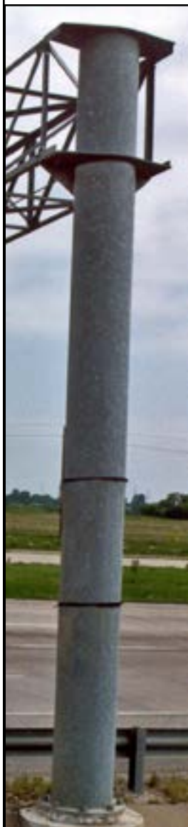
Galvanized sign structure
