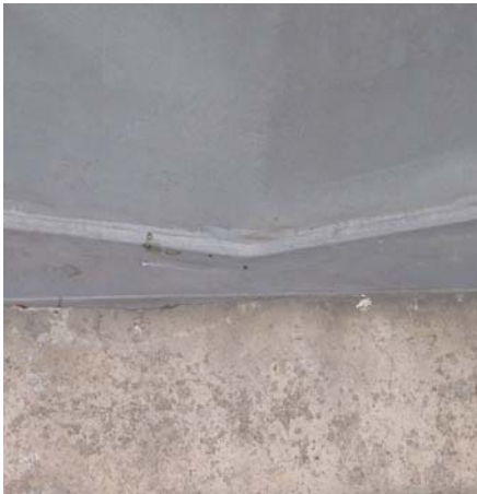
No corrosion products
