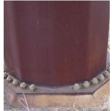
Weathering steel electrical distribution pole
