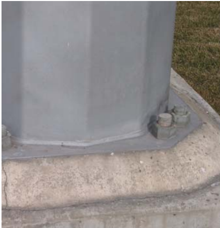
HDG steel electrical distribution pole
