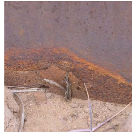
Significant corrosion products
