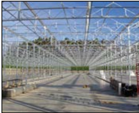
Metrolina Greenhouses Galvanized in 1971
