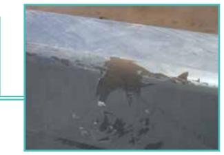
FIGURE 16: DELAMINATION (ACCEPTABLE IF MINIMUM THICKNESS LEVELS ARE MET)
