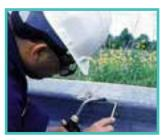
The final coating thickness for this repair must meet the specification requirement for the material category of the steel part being repaired with a maximum thickness of 4 mils (100  $\mu$ m). The thickness should be measured by any of these methods in A123/A123M that are non-destructive. Zincbased solder products closely match the surrounding zinc and blend in well with the existing coating appearance.
