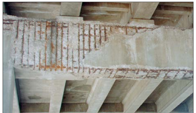
Corroded reinforcing steel caused dangerous spalling in the concrete on the underside of this bridge
