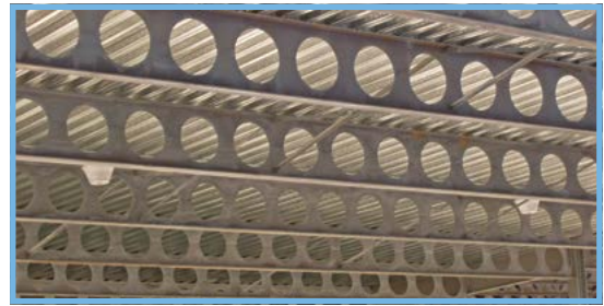
Arysley Parking Garage Charlotte, NC
