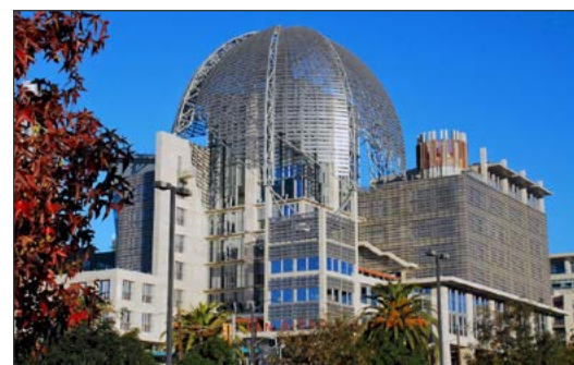
The San Diego Central Library utilizes galvanized steel for corrosion protection
