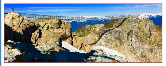
The Cloudraker Skybridge's walkway of galvanized steel grating and open mesh side panels allow adventurers to see the valley floor below. And the Raven's Eye Cliff Walk provides an unencumbered view on the cantilevered platform jutting out from the West Ridge.
