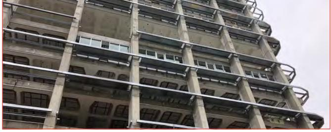
concrete, steel and glass while keeping the main support of the tower intact. Two additional floors were added, then the reconstruction of the exterior continued. According to the University of Calgary, "Unlike any other building on campus, MacKimmie Tower's double-skin exterior will respond to changing weather and work with the exposed concrete structure and mechanical systems to minimize energy use and optimize internal temperature, daylight, and air quality for occupants."
