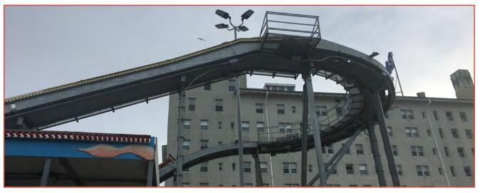
The High Seas Log Flume is vulnerable to the salt air and harsh weather all year around, and in addition to these harsh conditions, the ride uses chlorine water that is bad for carbon steel. After withstanding more than forty years of use and abuse, the owner wanted to utilize hot-dip galvanizing on the refurbishment of this timeless amusement ride.
