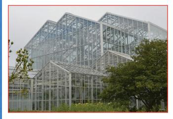
and coupled with concerns of corrosion of the pipe steel, came back to Michigan with the suggestion to utilize hot-dip galvanized steel. The rest of the brain trust agreed unanimously, so the design began with hot-dip galvanized steel as the coating of choice.
