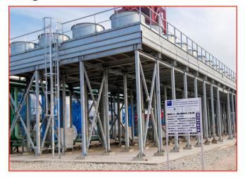
Acorn Infrastructure Services Unit 03 – 100 MW HFO Operated Power Plant residing East bank of the Karnaphuli River is now in operation and will operate throughout its contract period with minimal maintenance cost of corrosion thanks to the decision to use hot-dip galvanized steel.
