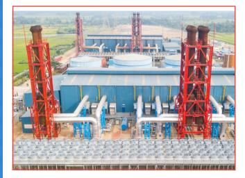
Acorn Infrastructure Services Unit 03 – 100 MW HFO Operated Power Plant is located in Jhulda, close to the port of Chittagong, Bangladesh. The Power Plant consists of 13.201 MW 8 units of ultra-efficient Caterpillar HFO Generator sets with combined capacity of 100 (± 10%) MW to supply to the national grid at Jhulda, Chittagong.
