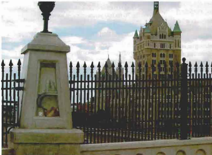
The Hudson River Way Pedestrian Bridge, a walkway over the Hudson River in Albany, N.Y., is a showpiece of powder coating over hot-dip galvanizing. The coating needed to withstand the elements of the Upstate New York climate, along with winter road salt and summer skateboarders. The handrails also feature powder coating over the galvanized surface. Hubbell Galvanizing of New York Mills, N.Y., powder coated the bridge, which was fabricated by Riverside Fab, Glens Falls, N.Y., and engineered by Clough, Harbour, & Associates, Albany, N.Y. The architectural firm was Einhorn, Yafee, and Prescott, Albany, N.Y. The design consultant firm was Carol R. Johnson Associates of Boston.
