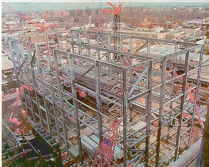
Fig. 1. Industrial plants can justify using hot-dip galvanized steel for external and internal structural elements because there are no maintenance costs.
