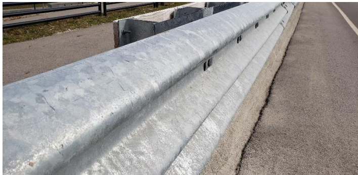
Figure 1: Natural Patina of Galvanized Steel
