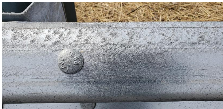
Figure 6: Natural Patina of Galvanized Steel Guardrail and Components
