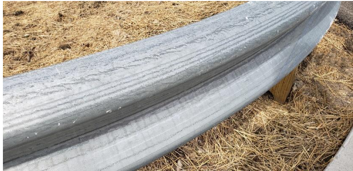
Figure 5: Natural Patina of Galvanized Steel Guardrail
