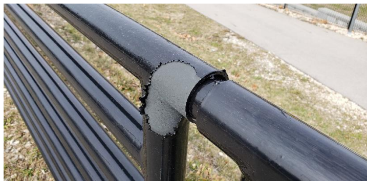
Figure 3: Paint Removed from Top of Rail
