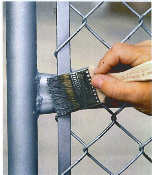
Zinc-rich paint application.
