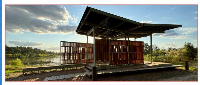
What truly sets this project apart is its thoughtful design informed by galvanizing. Architecture graduate students, after touring the galvanizer's plant, grasped the critical role of hot-dip galvanizing in ensuring the building's longevity and resistance to the elements. The design considered the intricacies of this coating protection, including scaling, venting, and drainage. Pre-welded assemblies were constructed before reaching the site, streamlining the on-site construction process.
