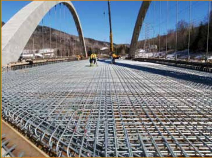
The suspended Stoneham Arch Bridge is an aesthetically pleasing solution to a unique site requirement. The choice of hot-dip galvanizing was preferred by the engineer because of its durability and cost compared to Cor-Ten steel in this highly corrosive environment. The resulting bridge is a beautiful and cost-effective marriage between structural steel and reinforced concrete.
