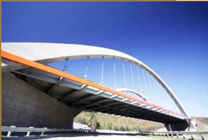
This type of bridge design, combining steel and concrete, is not often used. The unique design of this type of bridge makes it very interesting both architecturally and structurally. The use of galvanizing in all aspects of the bridge breaks new ground for our industry. Galvanized structural steel, galvanized reinforcing steel in the concrete, and even the supporting cables are galvanized.
