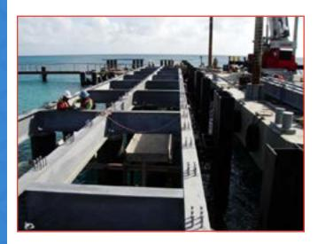
base of the new pier superstructure. As one last level of long-term protection for the pier's piling system, the pipe piles were coated with a coal tar epoxy.
