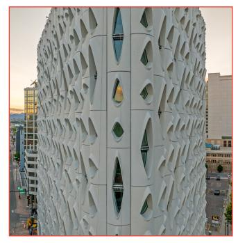
After considering other options, hot-dip galvanizing proved to be the best choice because of its sustainability, coating durability and corrosion performance over time. For the project owners, this was a no-brainer as they wanted a low-maintenance solution that wouldn't need constant repairs.
