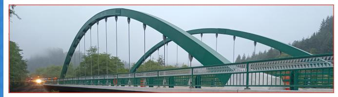
The Panther Creek Bridge, a 168-foot hybrid tied arch structure on U.S. Route 101 near Klamath, California, is a striking blend of engineering innovation and environmental sensitivity. Featuring galvanized steel arch ribs and floor beams, paired with post-tensioned concrete tie beams, it marks California Department of Transportation's (Caltrans) first-ever use of hot-dip galvanizing for primary structural components in a bridge project.
