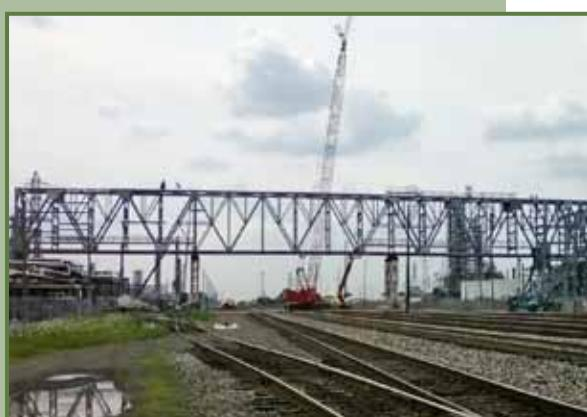
**S**panning eleven active railroad tracks, the Marathon Oil Bridge needs durable protection from the rough, corrosive industrial environment of the Detroit railway system. With a rigorous and intensive production schedule, the bridge was able to take advantage of the quick turnover provided by the hot-dip galvanizing process.
