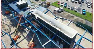
dip galvanizing would provide the necessary protection, but wouldn't match the desired color scheme. So, the team opted to use a duplex system satisfy all of their requirements.
