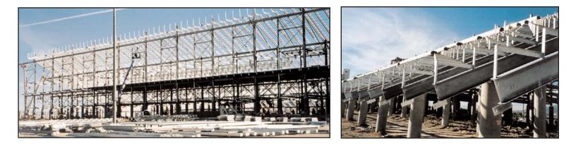
Hot-dip galvanized steel handrail, guardrail, stands, and fencing enjoys a long history of success in NASCAR circuit racetracks. This made the selection of zinc-coated steel for the Dale Earnhardt Terrace of the Las Vegas Motor Speedway an easy decision. A long-term, maintenancefree facility with an attractive appearance that is compatible with the rugged image of NASCAR racing, was a driving force in the decisionmaking process.
