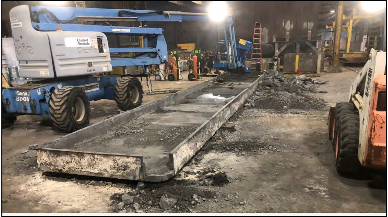
Kettle bottom almost cleaned ready to cut.
