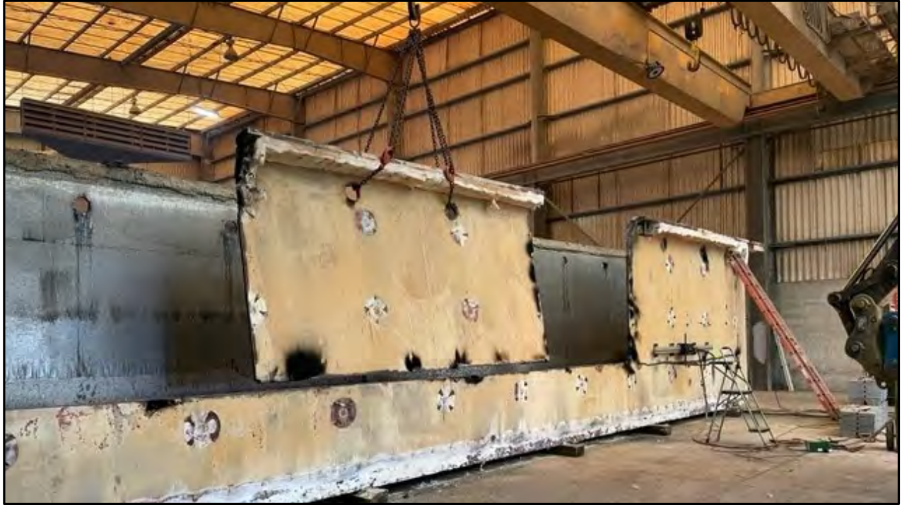
Removing manageable pieces of old kettle
