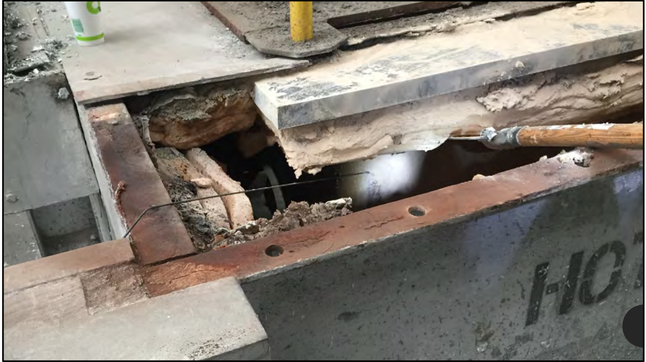
Another corner leak from not keeping walls clean.
