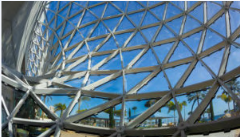
Fig. 6 Detailed look at the HDG steel support system
