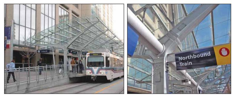
The City of Calgary, Alberta is a leader in the use of hot-dip galvanizing and duplex systems for infrastructure. Over the past decade, duplex systems have been used extensively on major overpass guardrails and pedestrian rails. Recently, the city specified hot-dip galvanized reinforcing steel in all bridges. So when the city was ready to refurbish the 7th Avenue Light Rail Transit (LRT) System, hot-dip galvanizing was the logical choice.
