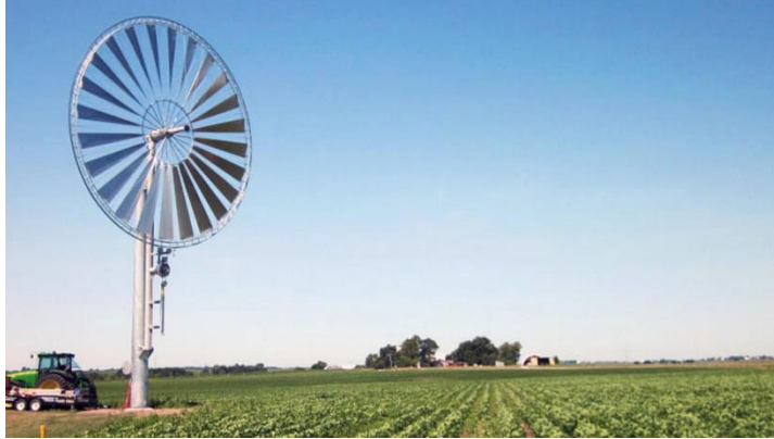
Fig. 5. Keuka Energy Wind Towers- Ainsworth & Fairfield, IA
