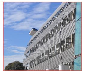
At night the point loaded, galvanized steel and glass-enclosed stair towers glow to create lanterns. Dynamic blue LED signal lights are programmed to chase around the helix. The decks feature an automated parking management system. hot-dip galvanized steel ensures all of the structures will remain a corrosion-free centerpiece of the airport landscape for years to come.
