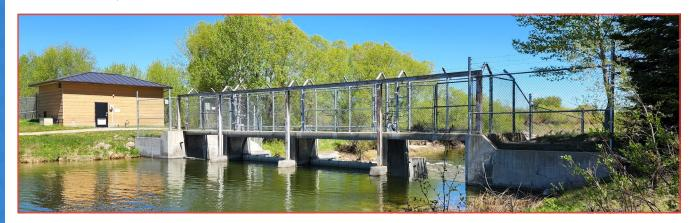
ot-dip galvanized steel proved to be the perfect solution for major upgrades to the Candle Lake Control Structure, located at a popular recreational site in Northern Saskatchewan. The structure regulates lake levels and controls discharges into the Torch River, ensuring both environmental stability and public safety.
