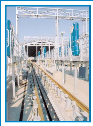
Built to service all 28 locomotives and 78 passenger cars that run on the Capital Corridor and San Joaquin lines for CalTrans, its new maintenance facility integrates maintenance-free, hot-dip galvanized steel into most facets of its design.
