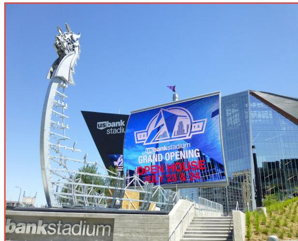
Due to the enormous size and configuration of the individual components, multiple facilities were called upon to complete the galvanizing of this structure. The contractor in charge of fabrication, coating and assembly of the structure worked hand-in-hand with multiple galvanizing facilities and designed the ornamental dragon head and mast components with best practices for hot-dip galvanizing.
