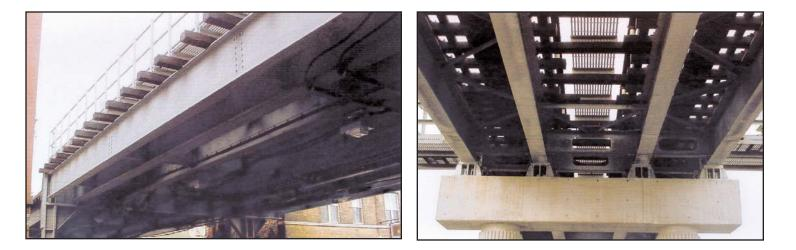
Comprised of 13,117 tons of hot-dip galvanized steel stringers — up to 66 feet in length, diaphragms, bearing assemblies, and top lateral beams, the Douglas Blue Line elevated structure is a 4.6 mile transportation hub winding its way through the neighborhoods of Chicago.
