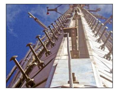
process. Because galvanizing is not a weather-dependent process, it can be completed year round without common delays. With quick delivery and fast installation, Pole-Max takes advantage of this benefit. Because Pole-Max is installed on galvanized monopole structures, the finish of the reinforcing channel closely matches the existing pole – and the protected steel will stand up to the elements for generations to come.
